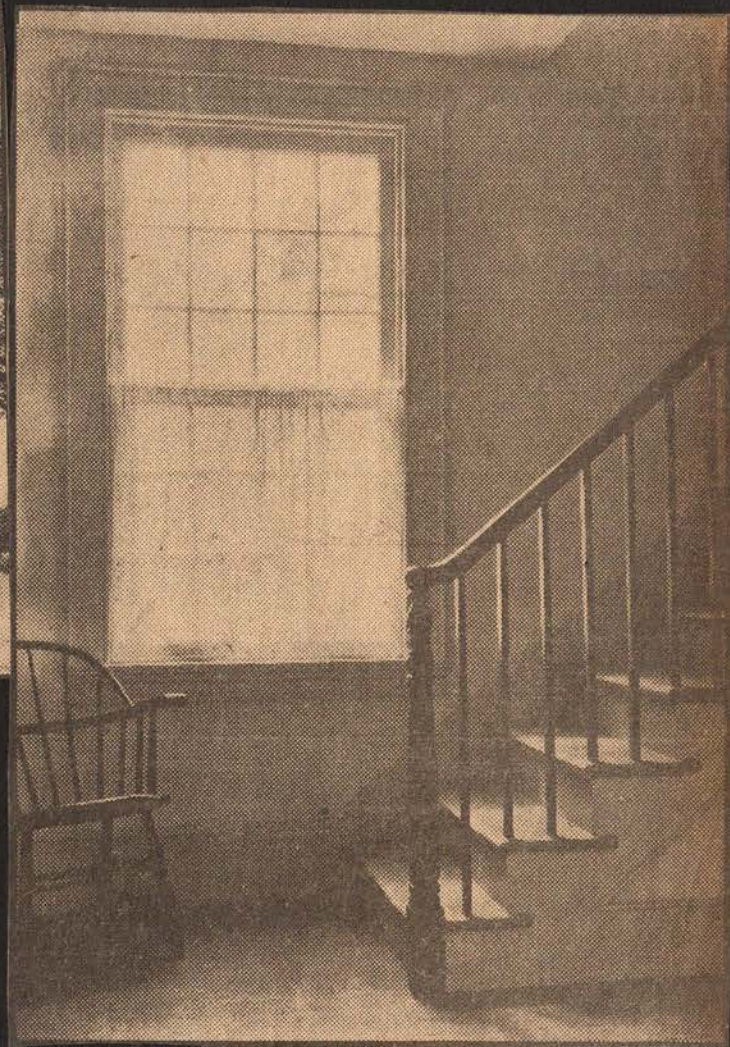
The Entrance Hallway
