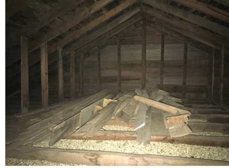
The house's asbestos-containing vermiculite insulation was abated in December
